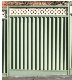
If a brick, stone, or concrete block wall is used for the required enclosure, no part of the wall may allow for finger, hand, or toe holds. The same restriction applies to any other type of material used for walls or fencing to enclose the outdoor area required at an ALF.
